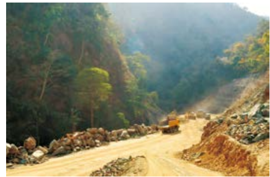
Fig. 6. Hydropower dam construction at Saw river (Mar. 4, 2014).
