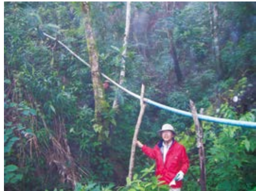
Fig. 8. PVC pipes are tied to tree or supported by forked branches to cross a stream (July 2007).
